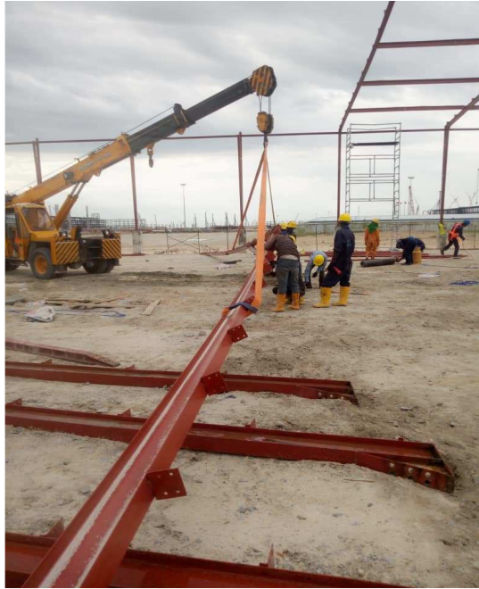
PLATE 2:- STEEL RAFTER BEAM READY FOR LIFTING
