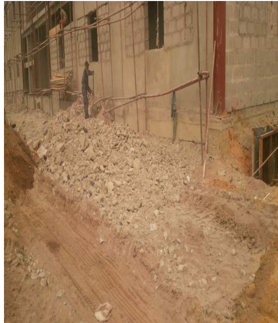
PLATE 6: PLASTERING WORKS ON BLOCKSETTING
