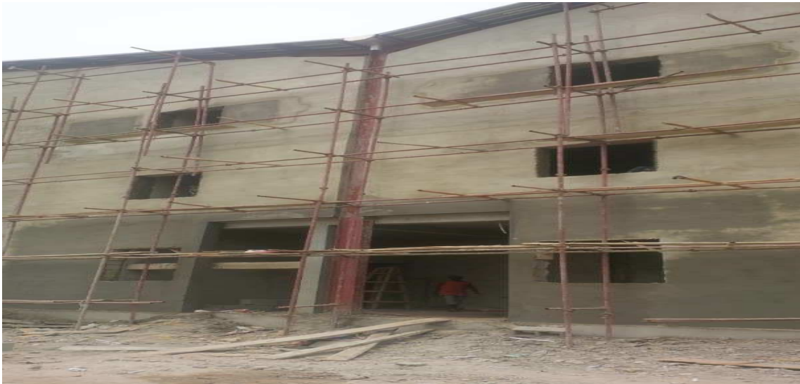
PLATE 8: PICTURE SHOWING COMPLETED & PLASTERED BLOCKWALL OFFICE AND WAREHOUSE FRAME
