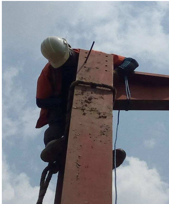
PLATE 4: CONNECTION OF STEEL RAFTER TO STEEL ANCHORION
