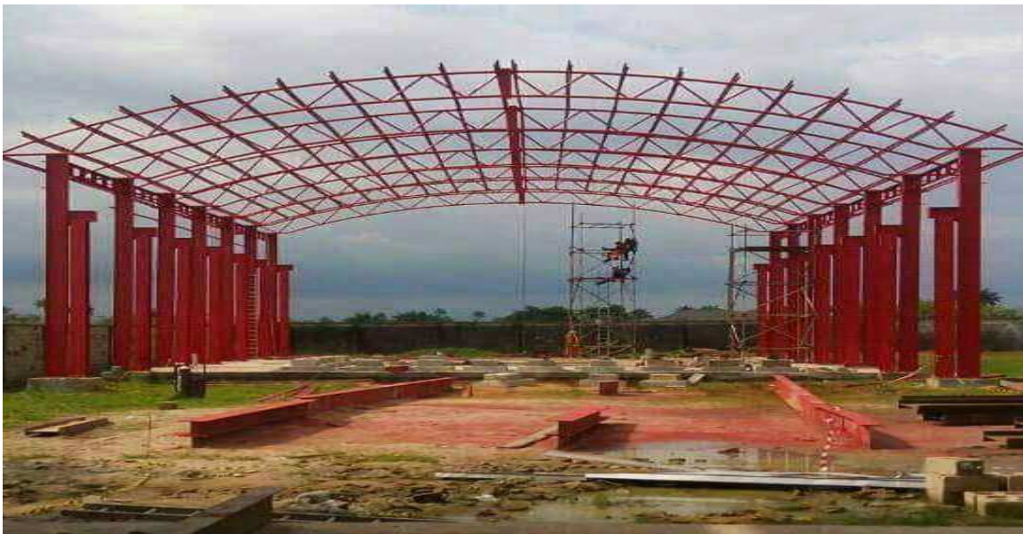
PLATE 2: COMPLETED STEEL PORTAL FRAME AWAITING ROOFING
