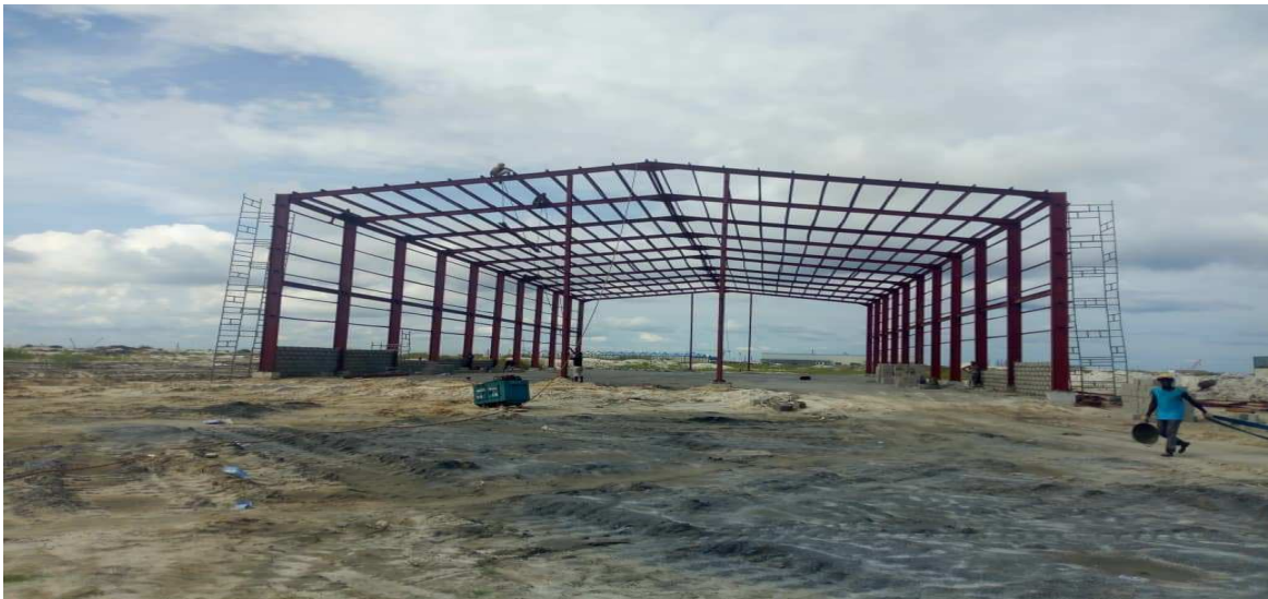
PLATE 6: COMPLETED STEEL PORTAL FRAME
