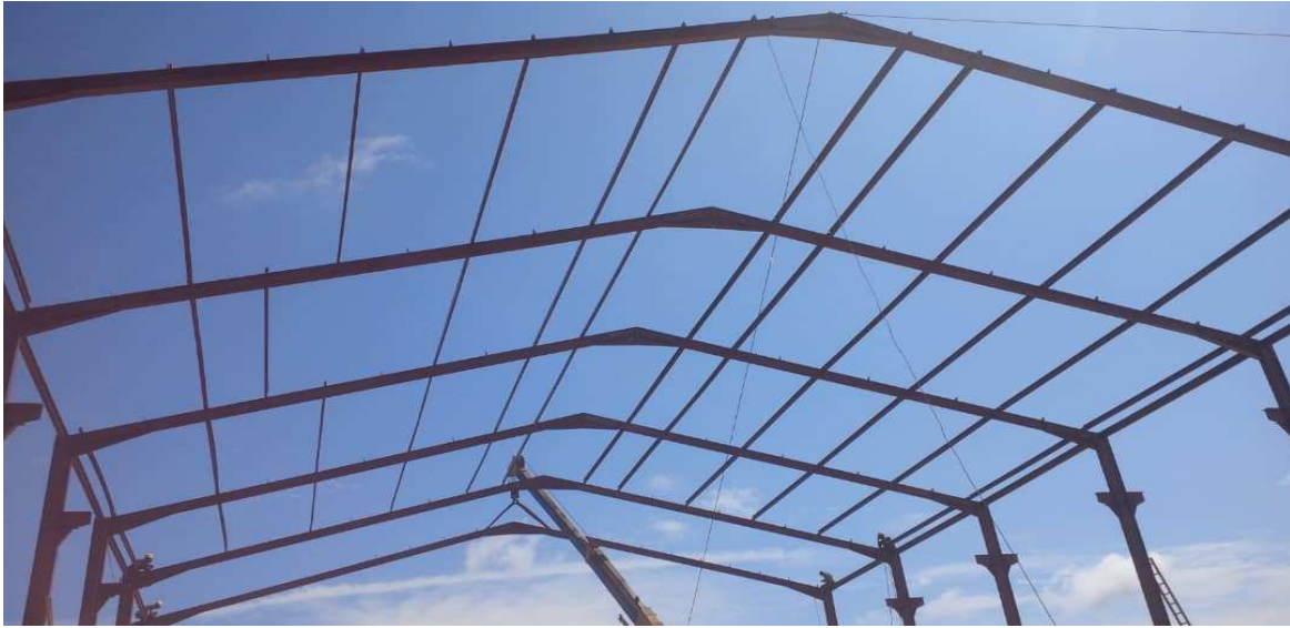
PLATE 5: ERECTED STEEL FRAME WITH ONGOING END CONNECTIONS
