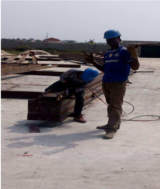
PLATE 1: FABRICATION WORKS ON STEEL RAFTER BEAM
