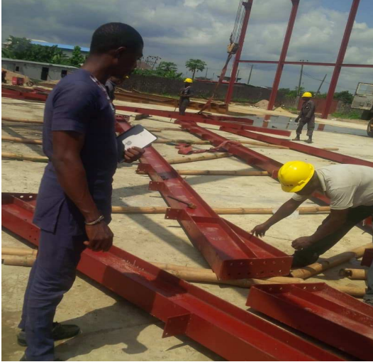
Plate 1:- Ongoing Fabrication & Assembling.
