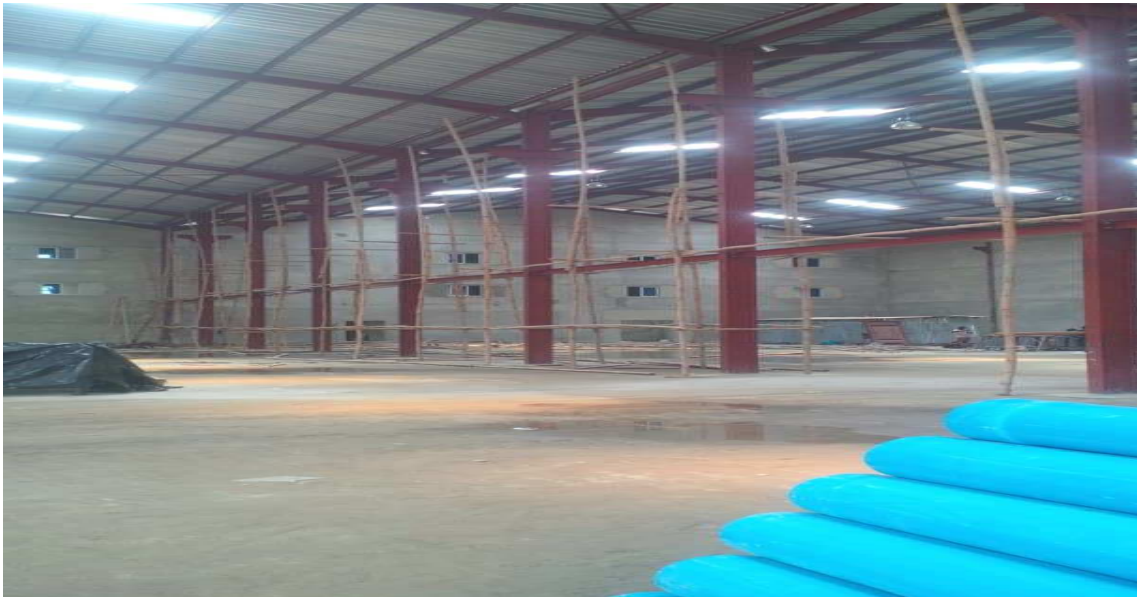
PLATE 7: PICTURE SHOWING INTERNAL STEEL FRAME OF WAREHOUSE AREA
