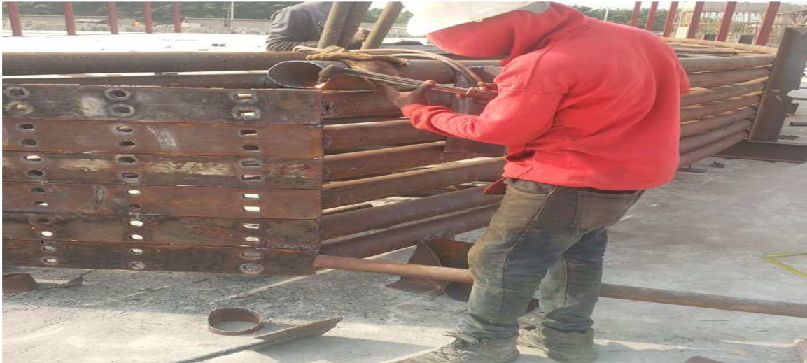
PLATE 1: ONGOING TRUSS FABRICATION WORKS
