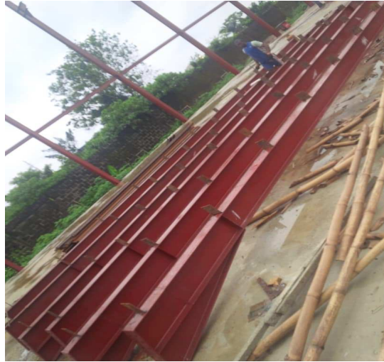
Plate 2:- Completed Steel Rafter beams.
