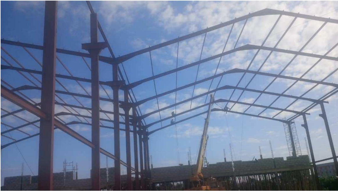
Plate 3: Ongoing Erection works and connection of steel rafter beams.
