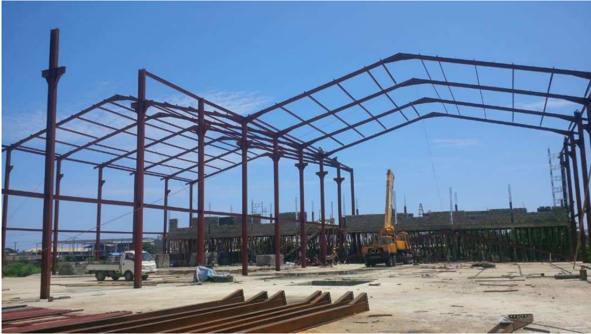
PLATE 4:- PICTURE SHOWING ERECTED STEEL FRAME
