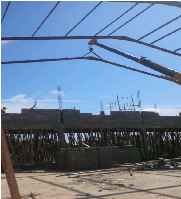
PLATE 5: ONGOING BLOCKSETTING AT OFFICE AREA
